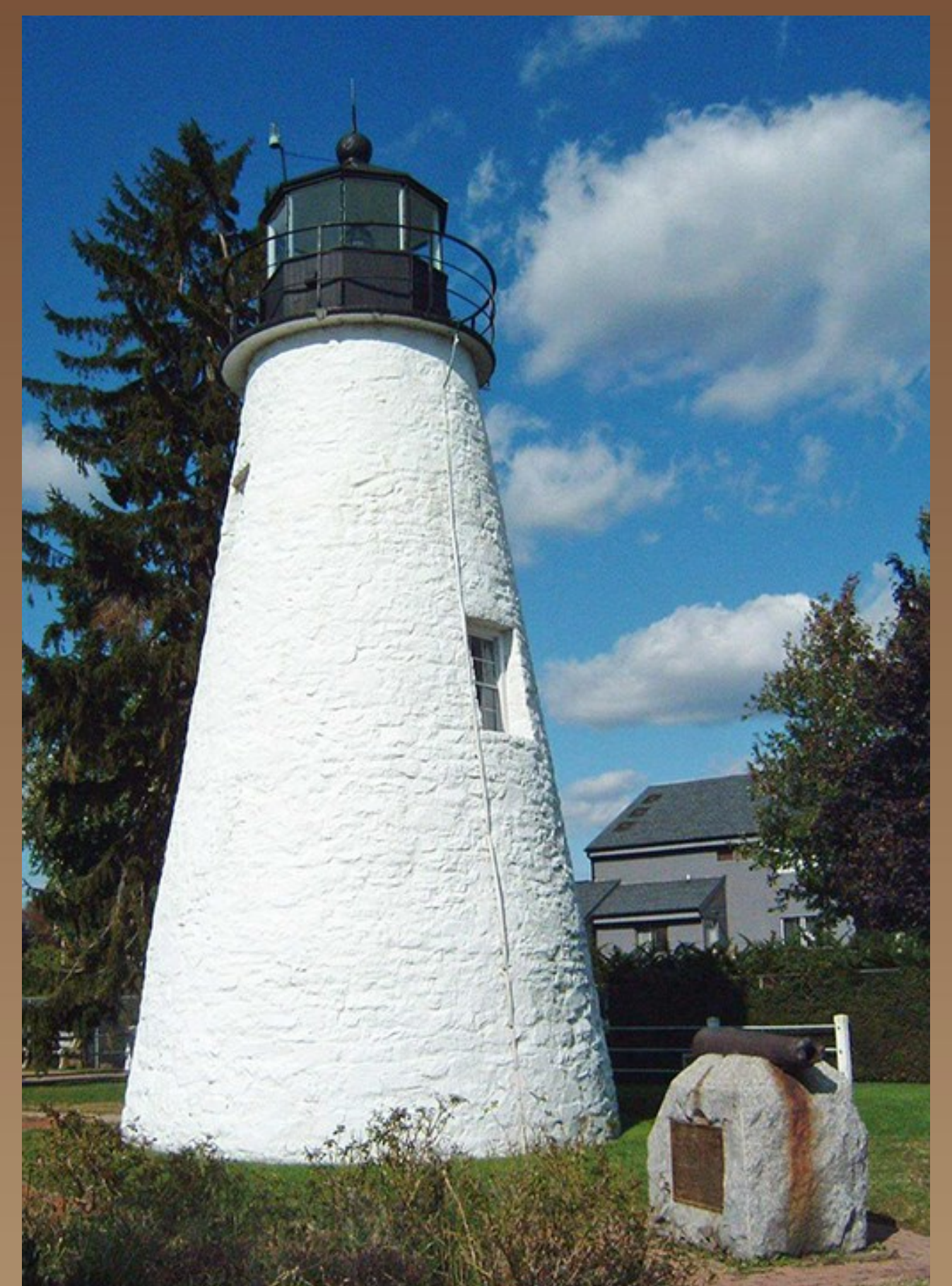
Figure 4 - John O'Neill memorial at the Concord Point Lighthouse prior to conservation.
